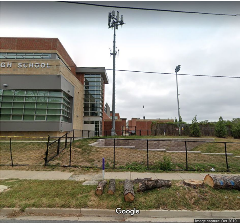
Wheaton High School, Montgomery County Maryland
