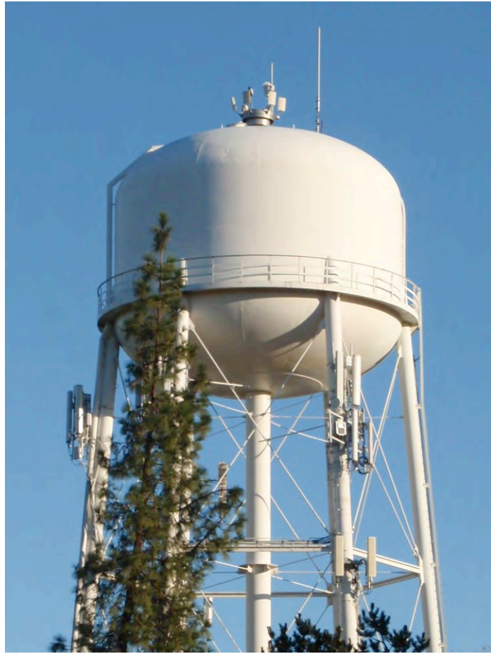
Davis water tower on Eighth Street near Elmwood Drive, November 2018. Two omnidirectional whip antennas and several smaller antennas are located on top of the tower. Numerous panel-style (sector) antennas are located below the tank, on the tower's sides.
