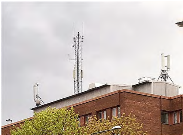
Figure 2: The case study location – several mobile phone base station antennas and TETRA antennas on the roof.
