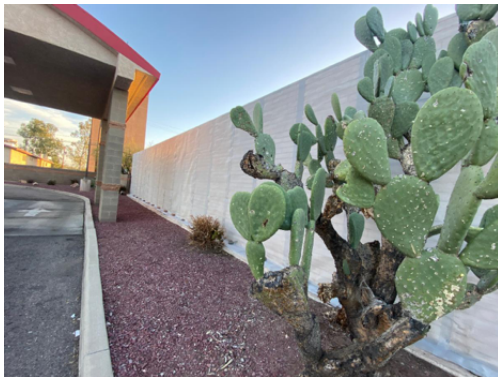
120 foot external wall covered with aluminum metal mesh screening
