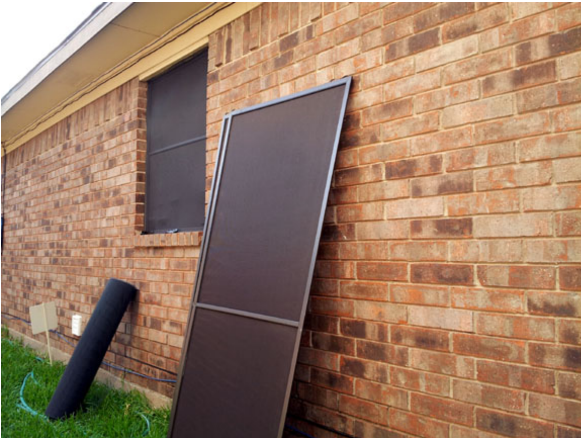
Covering entire windows and doors with aluminum screening only slightly reduces 24/7 rf entrance into home.
